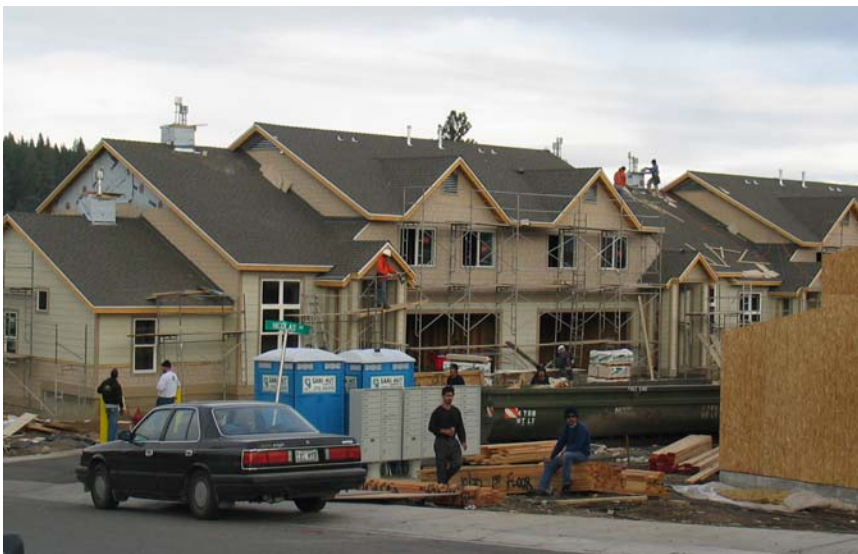
Construction activity can be a significant source of community noise.
